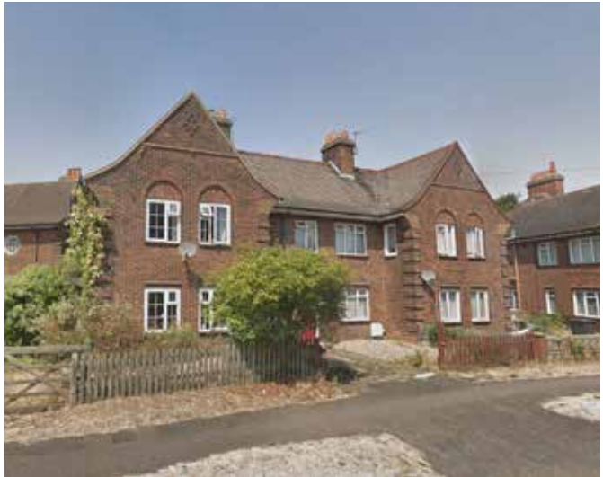
Early buildings in Shortstown resembling Arts & Crafts Movement aesthetics
